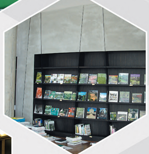
Interior Wall SCG Experience, Bangkok Using SCG Smartboard Square Edge 8 mm. thick plastered with plastering cement, make 1 - 3 cm. skim coat.
