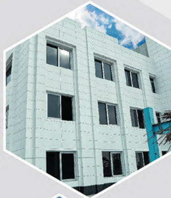
Exterior Wall (Iran) SCG Smartboard 1.2 cm
