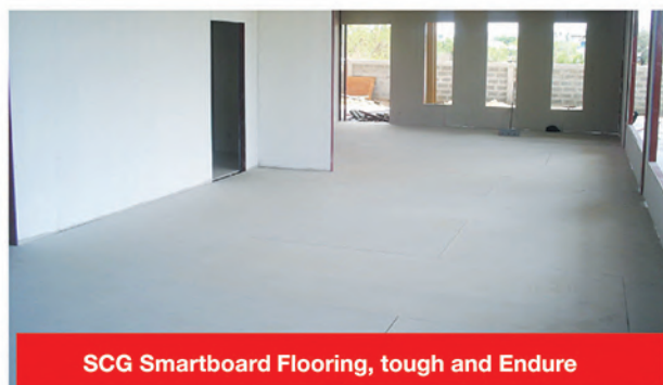
SCG Smartboard Squared Edge 16, 18, 20 mm. thick
